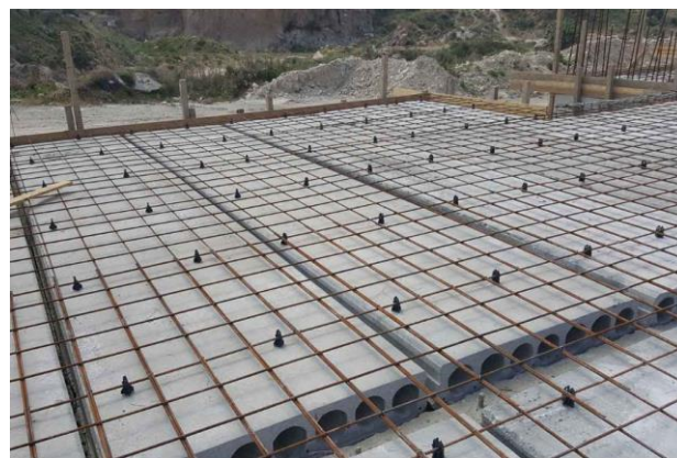
Figure 5 Typical Hollow core slab construction
