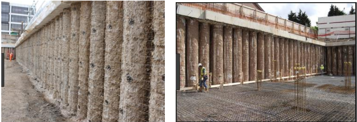
Figure 8 Embedded Piled Wall
