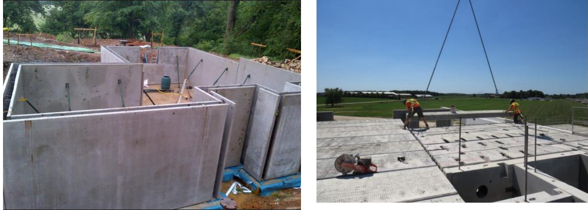
Figure 4 Typical twin precast concrete wall system and hollowcore slabs
